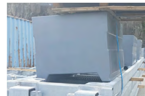
Pontong under montering
